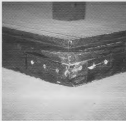
Figure 10b: Detail of corner with L-shaped bracket removed.
