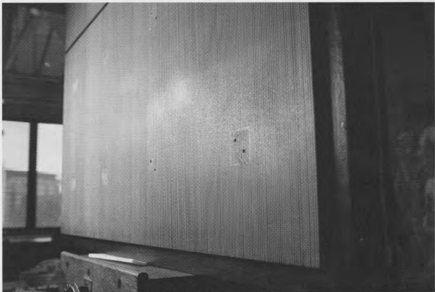
Figure 13: Detailed of the cleaned areas and the difference in gloss.
